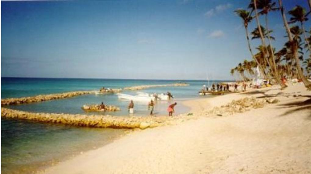
**Figure7. Rock placement on top of Reef Ball breakwater and connected to shore.**
