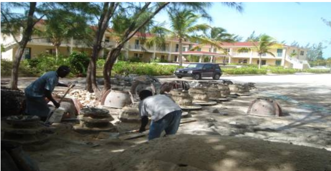
Figure 3. Early fabrication stages.
