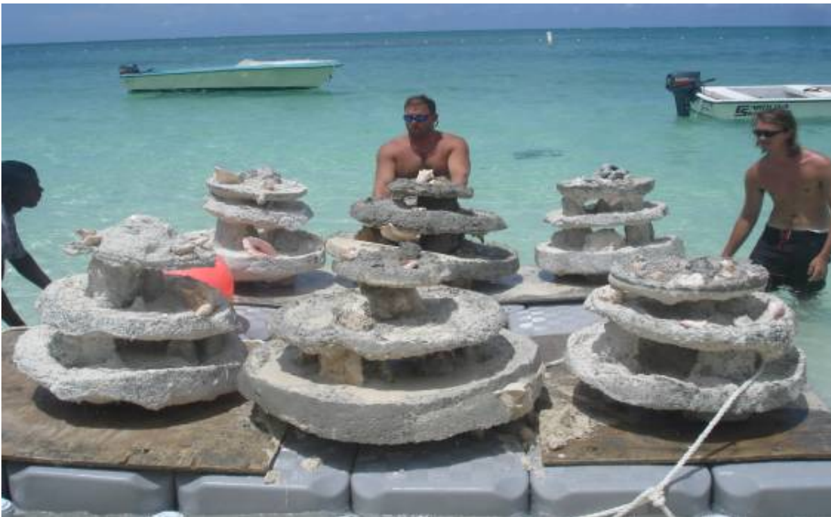
Figure 5. Transporting modules to site.
