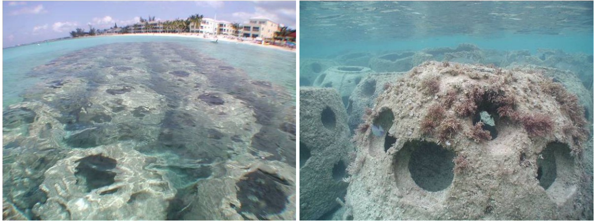
Figure 7. 5-Row Reef Ball Submerged Artificial Reef Breakwater offshore Grand Cayman
