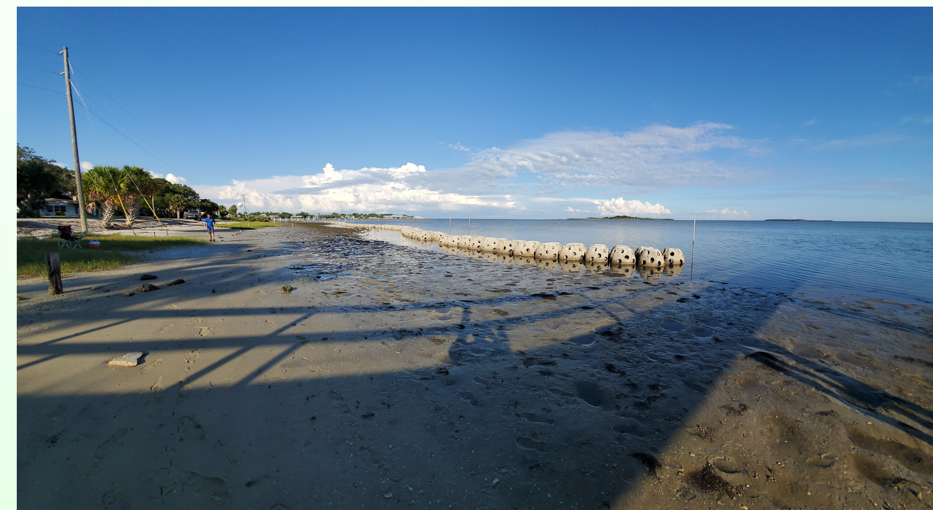
Reef Ball™ breakwater Airport Rd Cedar Key in 2020. This was designed to protect the road, homes and enhance the habitat for marsh grasses and oysters.
